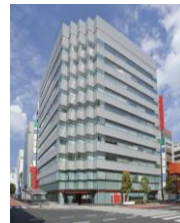
NRE Ueno Building
