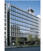
Former NOF Tameike Building
